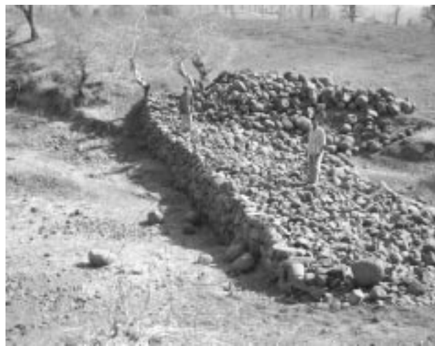
Gully bund to prevent soil erosion in the village of Juna Mozda, Gujarat
