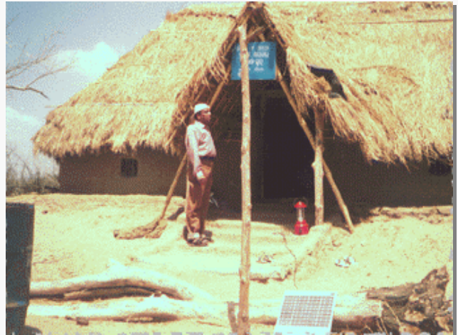
Mamta Grha (home of compassion), one of the many set up by the government to house destitute women and children temporarily, in the most ravaged regions
