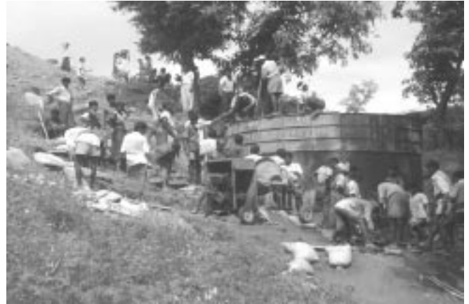
Village volunteers construct the check-dam in Bilgaon.
