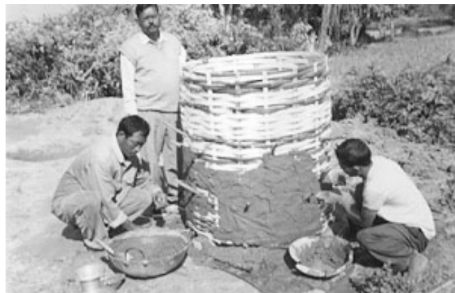
Construction of toilets in Dharikathi village, Assam.
